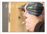
Once you have marked everything up drill a hole that goes the complete way through the door as in this how-to we will be using male to female bolt through fixings. Wood screws can be used just no need to drill all the way through the door. The boltthrough fixings give a much better result.
