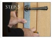
When you are happy with the fitting of both handles and the spindle length it is time to begin fixing the handles in place.
