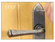
The male/female fixings will probably need to be cut down to size depending on the door thickness. This can be done by eye. Simply offer up the bolts to the edge of the door, taking into consideration the thickness of the handle backplate, and cut with a hacksaw down to desired length. Fix with a screwdriver each side of the door.
