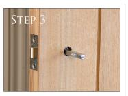
The spindle provided is designed to be used with a range of door thickness's so you may need to adjust the length depending on your door. You can check this by fitting the second handle to the other side of the door and seeing how much (if any) spindle is spare (still showing). Measure this amount and go to step 4.
